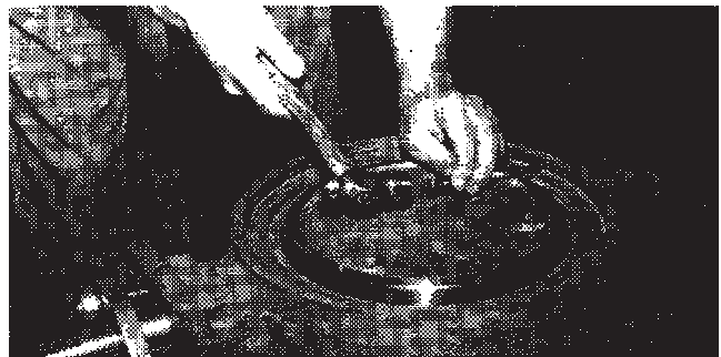
Tapping End Of Spring Into Body
