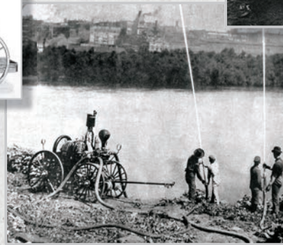
Pump testing on the Mississippi river near the factory.
